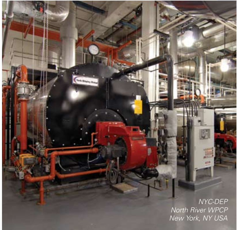
Series 500C Dry-Back Packaged Firetube Boiler
